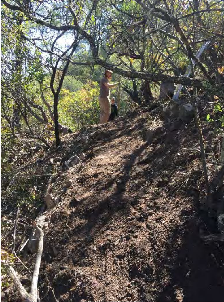
Figure 6.2a. Cutting trail for the GPR transect. Notice the angle of the hillside and trail. There were also several large rocks that needed to be removed to ensure a smooth and flat transect. After 8 hours of work, the slope over most of the 18 meter long transect was reduced to 10-20 degrees.
