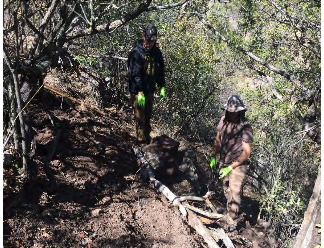
Figure 6.2a. Cutting trail for the GPR transect. Notice the angle of the hillside and trail. There were also several large rocks that needed to be removed to ensure a smooth and flat transect. After 8 hours of work, the slope over most of the 18 meter long transect was reduced to 10-20 degrees.
